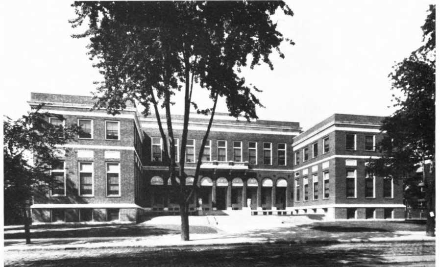
Figure 2. The newly completed Rochester Dental Dispensary in 1916.
