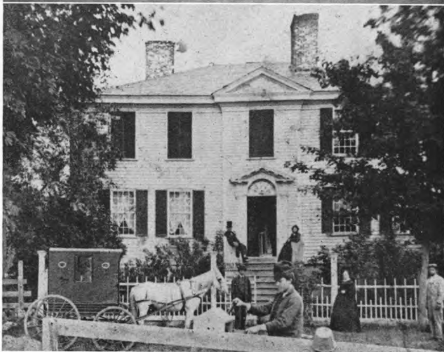
Top—Horace Wells' home at Westminster, Vt. Bottom—The home of Horace Wells' stepfather, Abiather Shaw, Jr., in Westmoreland, N. H. Both these houses are still standing and occupied.
