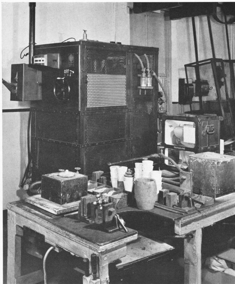
FIG. 1. High-frequency induction-furnace used in preparation of many alloys. Melts may be made under vacuo or under any gas.
